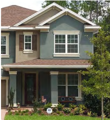
Columns should have been painted the trim color and not the body color. Don't confuse the material (stucco) with the architectural element.
