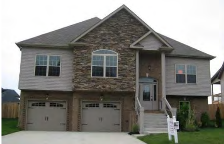
A rocket ship entry, columns that are too skinny and of stone used like paint – not allowed.
