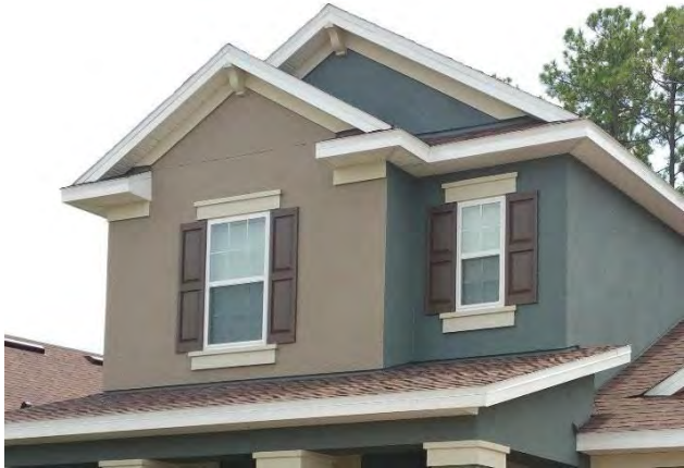
This is an example where the color ends on an outside corner.
